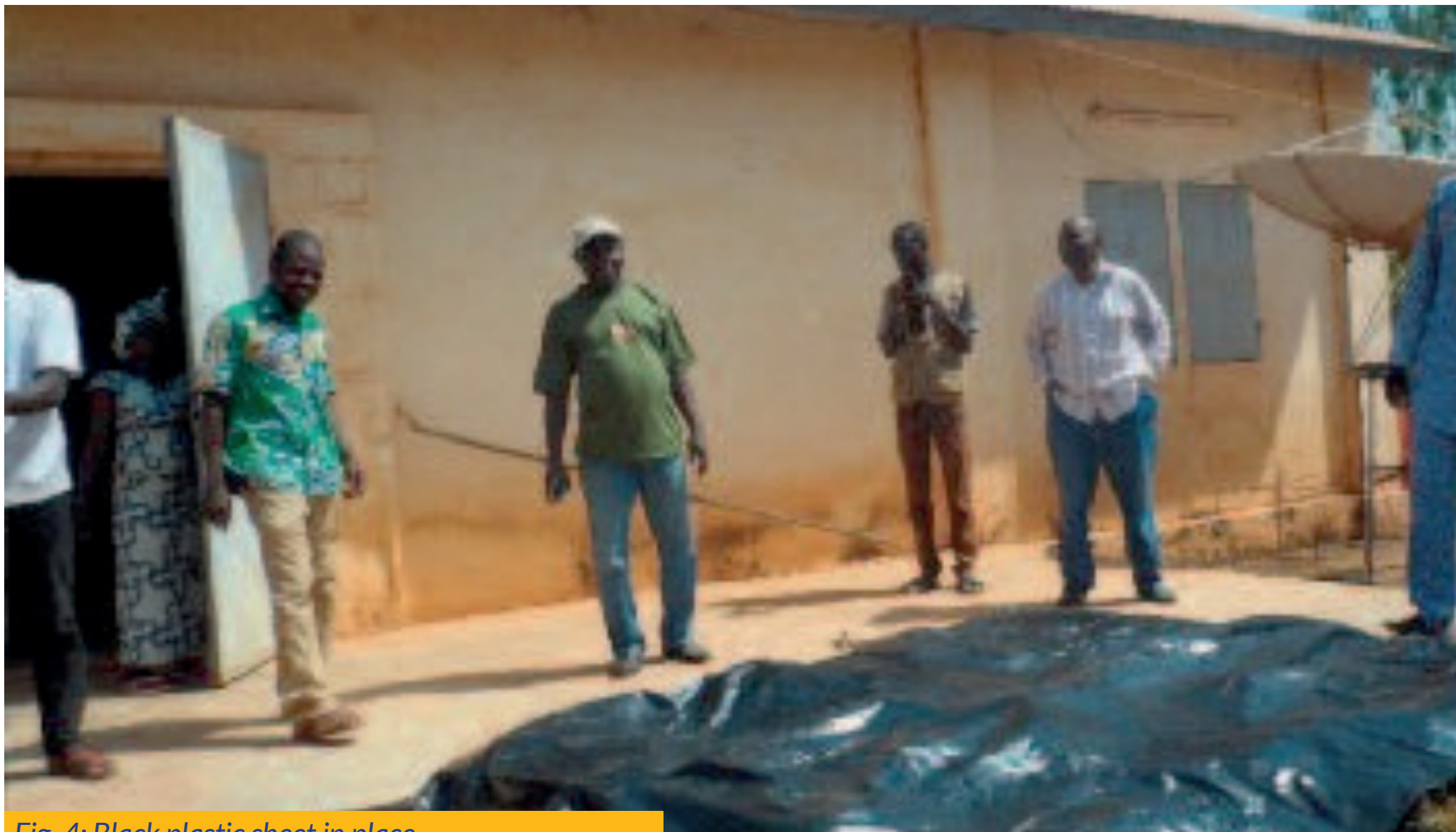
Fig. 4: Black plastic sheet in place
